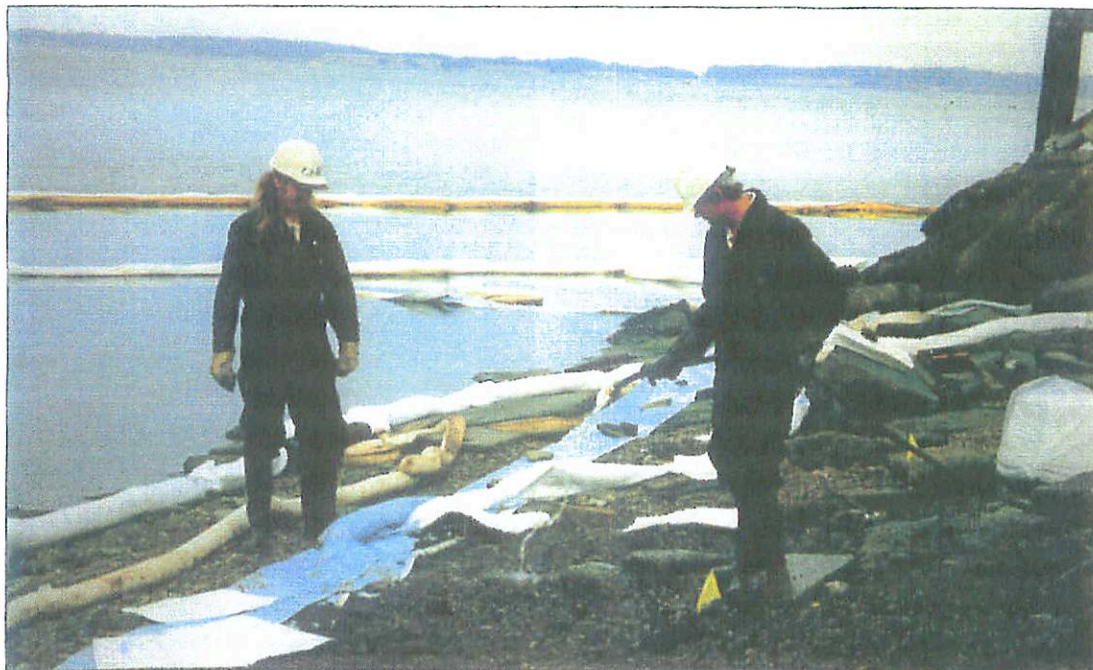
Figure 4 Field trial of CytoSol biosolvent application to release trapped oil from an oiled gravel beach on San Francisco Bay (November 1995)
